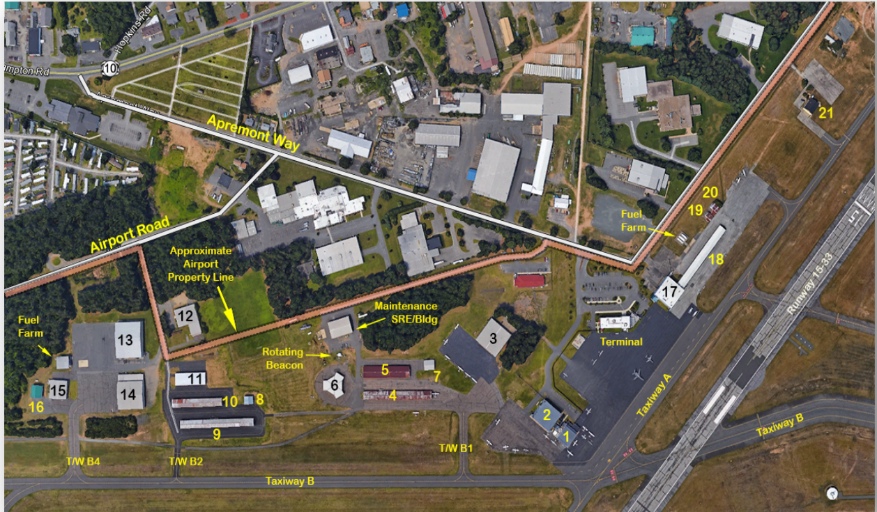
Figure 2.8 - BAF Civil Hangars
